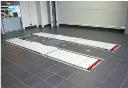
Level workshop floor
