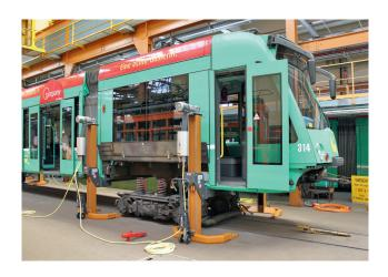
A special wheel engaging column lift solution for trams was designed for the Basel transport authorities (Basler Verkehrs-Betriebe). This challenging project was implemented by MAHA's Swiss-based partner, KSU/A-TECHNIK AG.
